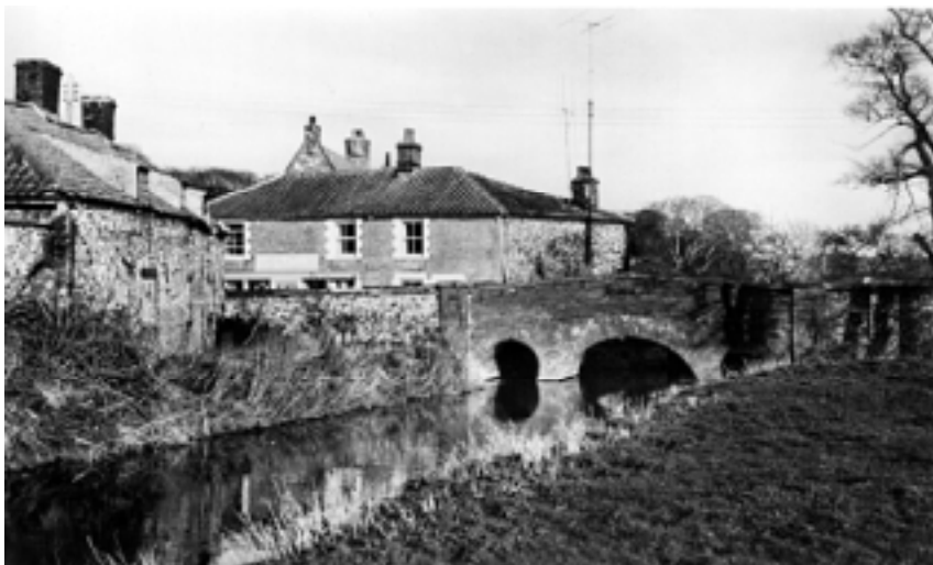
River Stiff and Stiffkey Bridge
